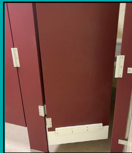
Bathroom stall modified to ensure more privacy for student with dwarfism
